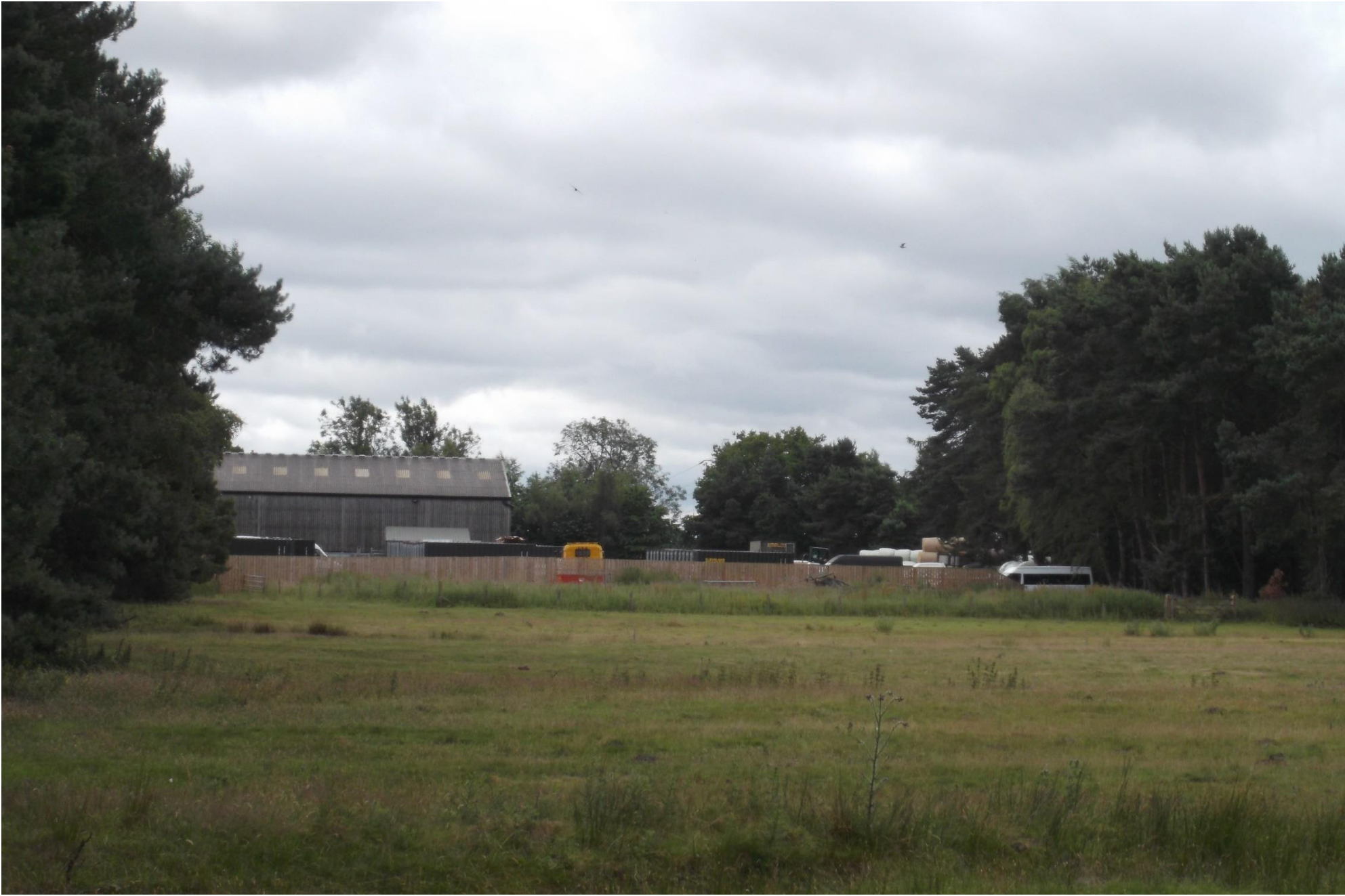
Exterior View from East
