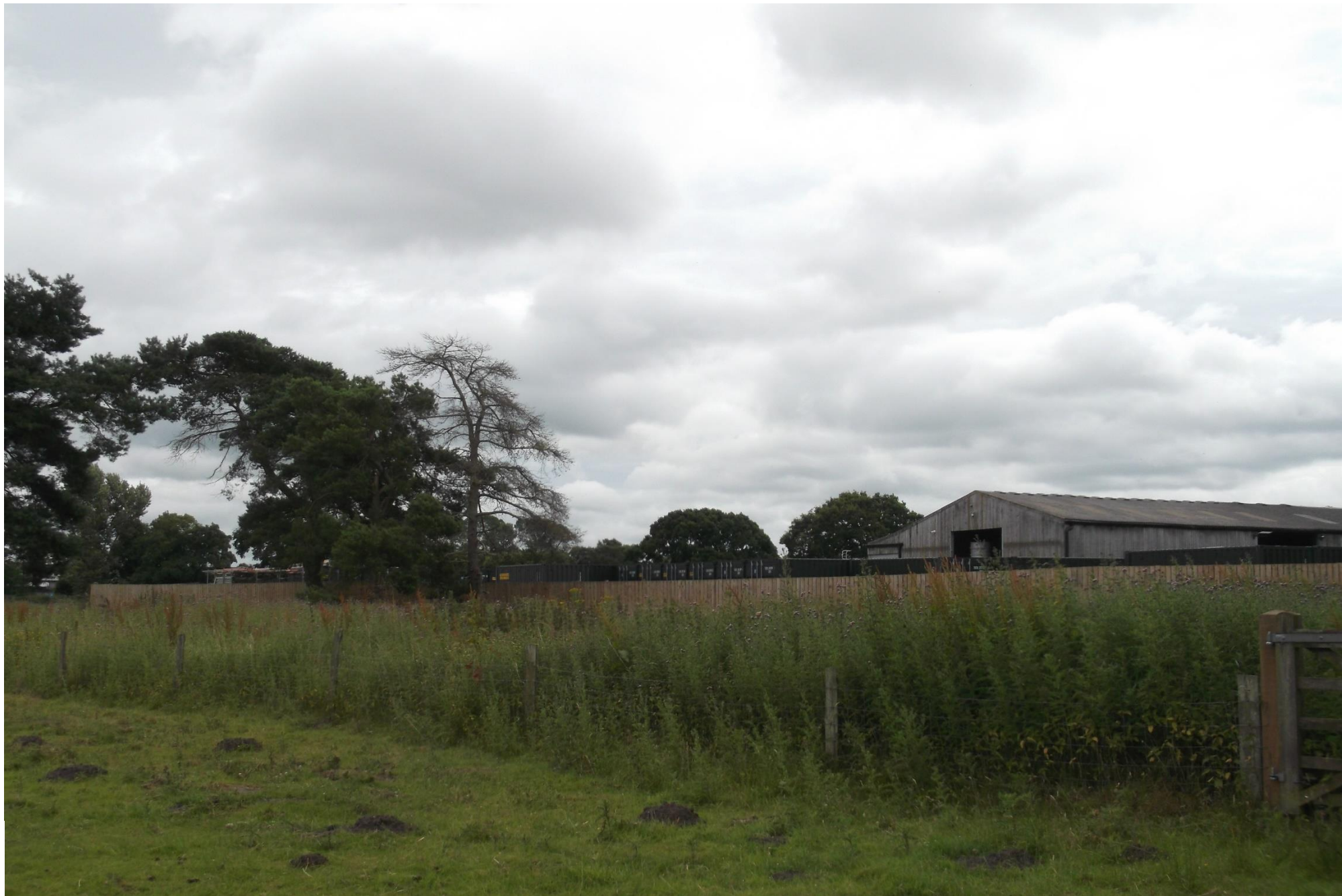
Exterior view of Site from Towthorpe Road (South)
